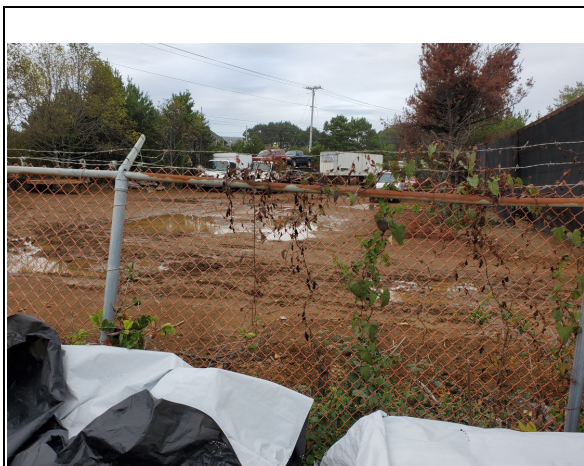
Photo 1: View from Copeland Lumber Company property line. Adjacent property recently purchased and
